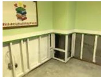
Over the next few weeks new wallboard and plaster will be installed, with a chair rail at the intersection of the old and new. After that new flooring will be installed.
